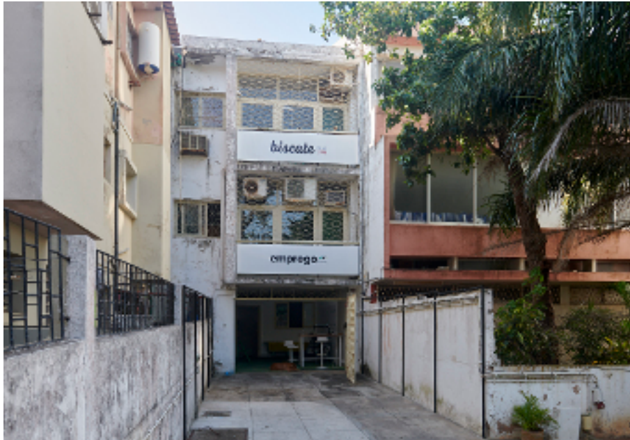
The UX office building in Maputo.
