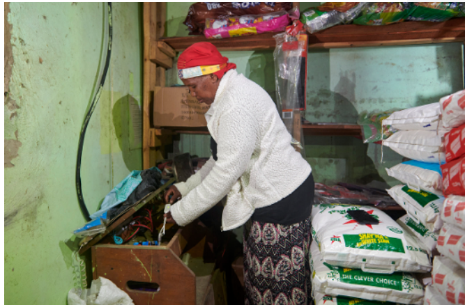
Sigcau checks the cable connections and the batteries.
