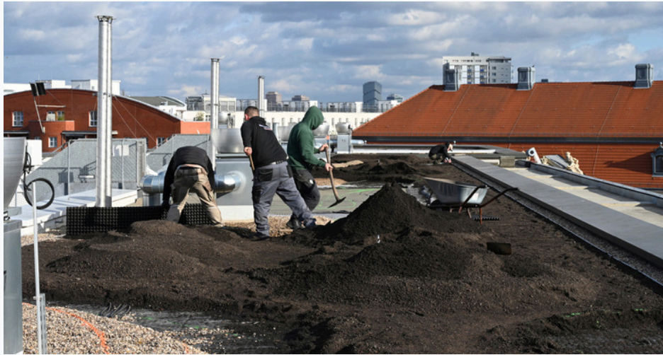
Rainwater can be collected with a layer of gravel and soil. © IBeB
