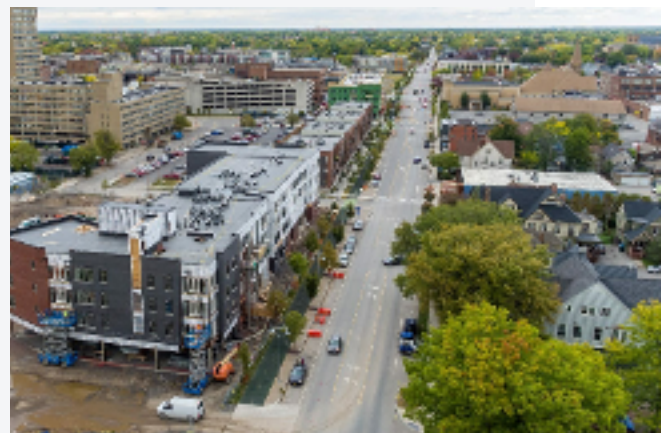
After: The new homes on the former freeway site under construction.
