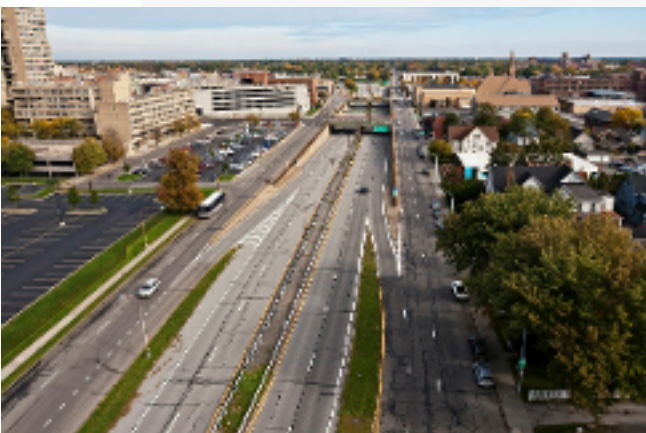
Before: The eastern Inner Loop before demolition.
